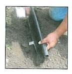
**Step 5:** Sink stake through the fin every 5 feet at a 45 degree angle
